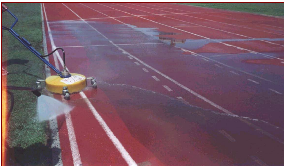
Washing of track to be done with rotary cleaning head & hand held pressure cleaner
